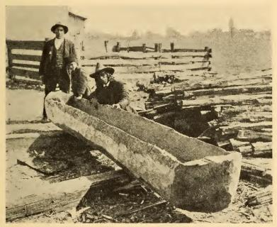
Fig. 77.—Dugout canoe of the Pamunkey in course of construction.
